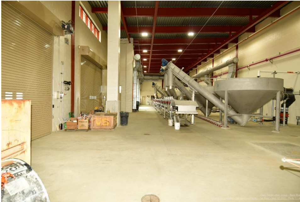
Back River WWTP Headworks Project – Grit Removal Facility; June 2021
